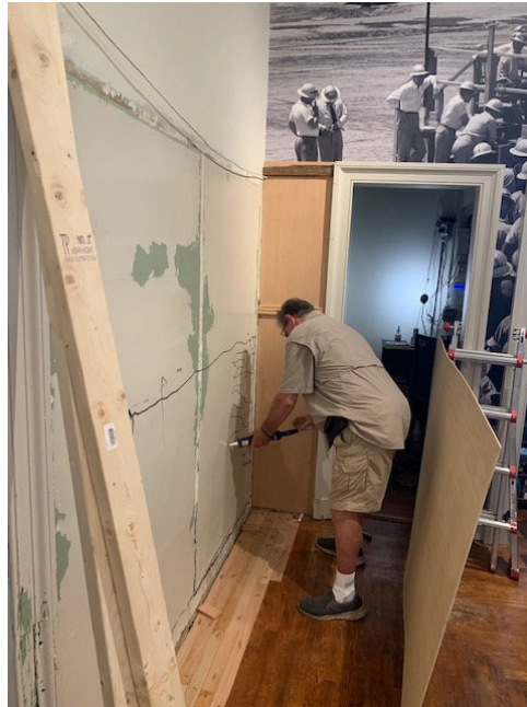
(Image 1) The bookshelves behind the docent desk have been removed. Here, Rex Nordeen applies glue to the wall in preparation for the wooden panel that will be added.
