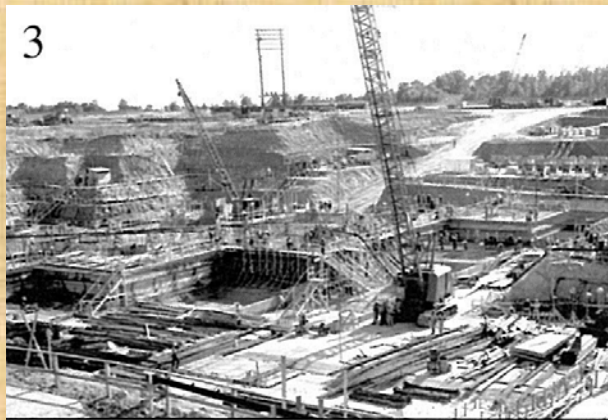
R-Area reactor building takes form at the base of the excavation
